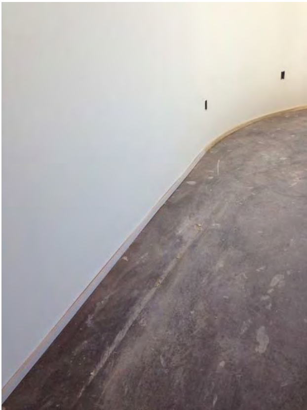
Drywall finish at curved wall
