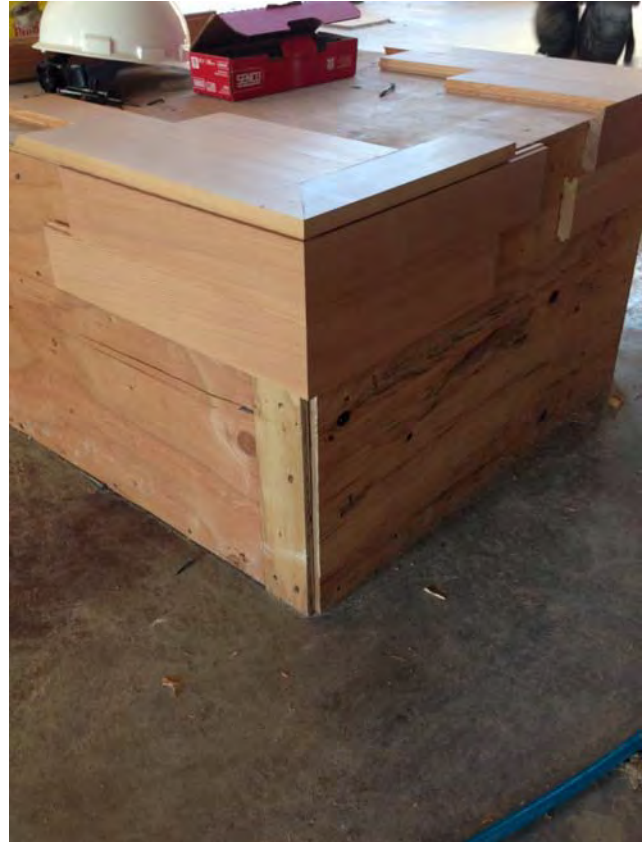
Mock-up of atrium stair finish sample
