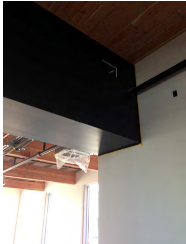
Paint begins at second floor
