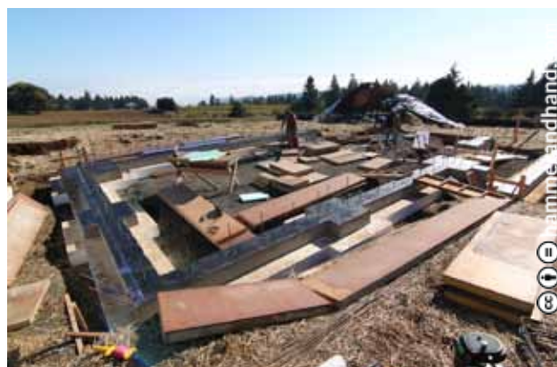
FOOTINGS AND STEM WALL COATED WITH CAPILLARY BREAK/FLUID APPLIED WATERPROOFING.
