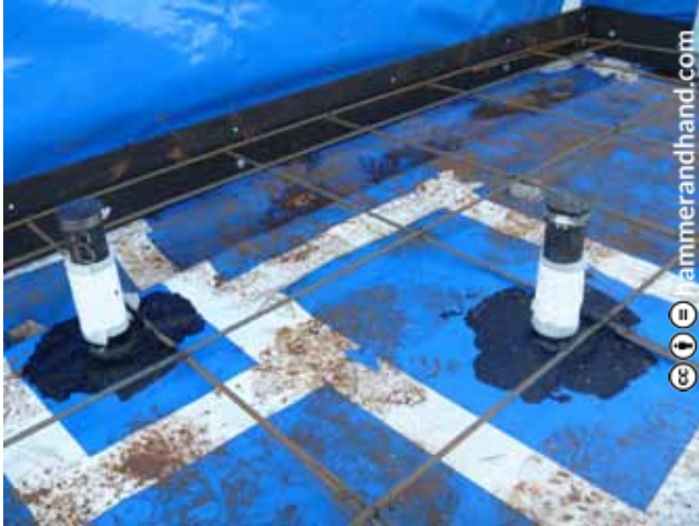
TAPED SEAMS AND SEALED PENETRATIONS IN THE SUB SLAB VAPOR AND SOIL BARRIER.
